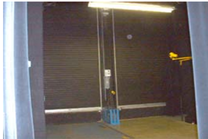
View of the loading dock from inside the backstage. Note the power lift at the left door.
