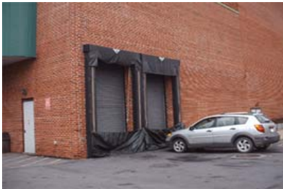
The Arts Center's double loading dock is located directly off the stage and with clear access for backing large rigs in from the street to the dock portals.
