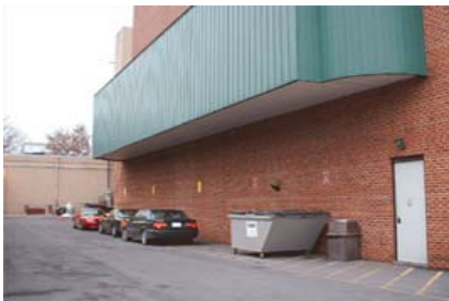
Space is available under the overhang area for four buses or trucks.
